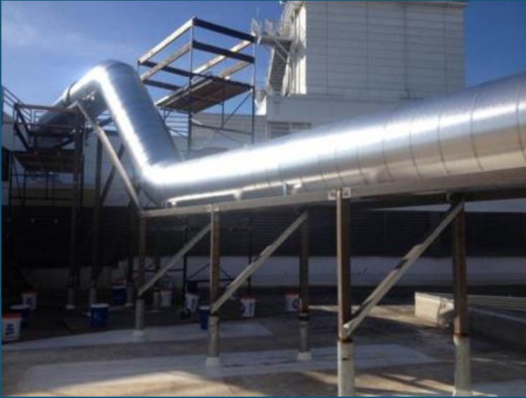
2 nd Floor Mezzanine Infrastructure Upgrade
